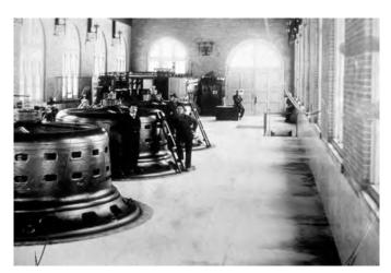
Trenton Falls Hydroelectric Plant, West Canada Creek, Located at the bottom of a dramatic gorge and normally off-limits to the public, the Trenton Falls plant had the highest head reaction turbines in the country when it was completed in 1901. The original plant and its 1914 addition remain in operation today, largely unchanged after a century.
