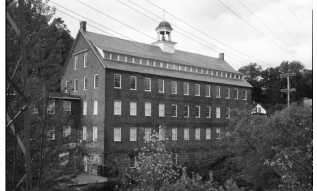
American Precision Museum (1846) originally the Robbins & Lawrence Armory. Jet Lowe, HAER.
